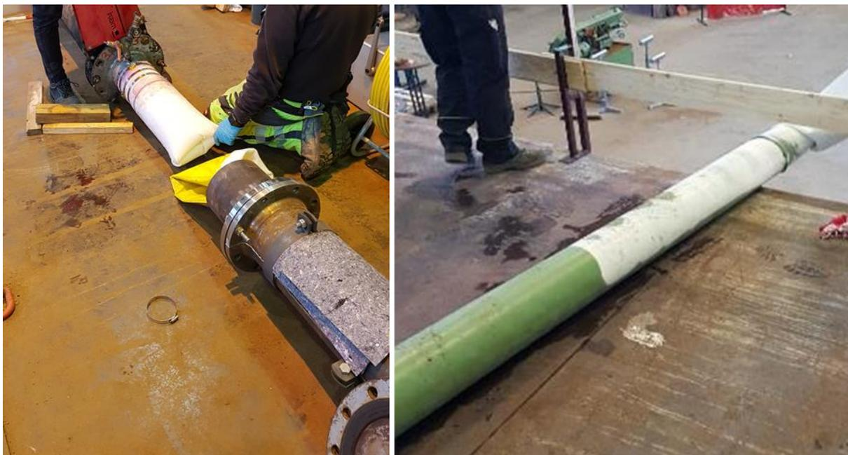
Figure 38. Pull-in and inversion process: "SaniPipe"(left) and "Esders HPS Liner" (right).
