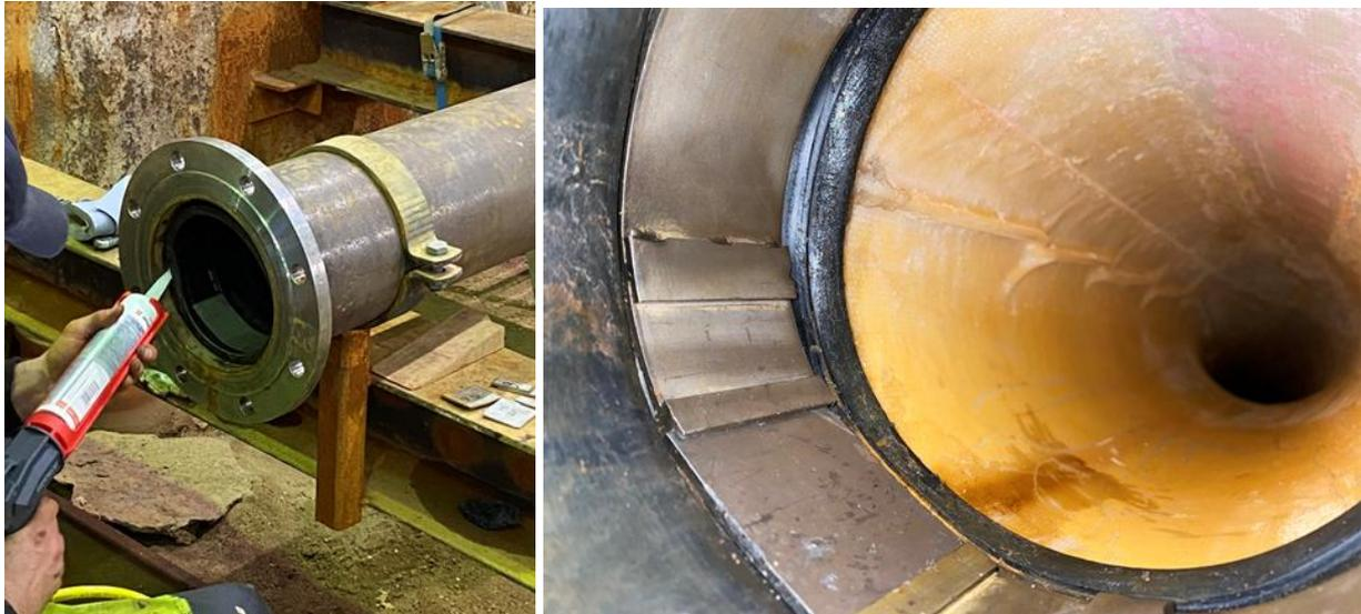
Figure 17. Replacing the sleeves with acetate silicone with "SaniPipe": applying the sealant (left), rework result (right).
