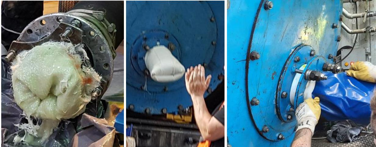
*Figure 39 Inversion method: "Starline Structure-S" (left), "Nordiflow W PE" (middle/right)*
