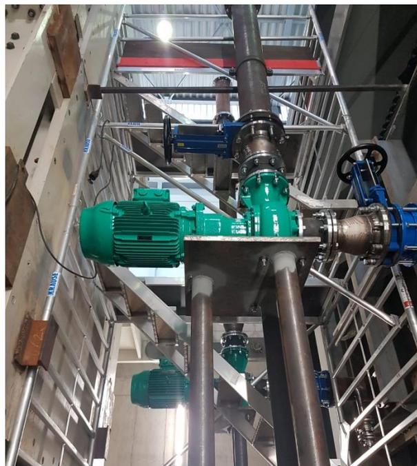
Figure 8. View of the two pumping stations, showing for the nearer pump its support platform, riser pipe with gate valve (leading upwards) and suction pipe coming from the right, also with a gate valve.
