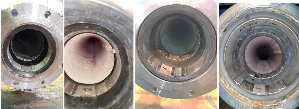
Figure 41. Liner end sleeves from left: "Starline Structure-S" (Kempe), "SaniPipe" (Amex), "Esders HPS Liner" (Amex) and "Nordiflow W PE" (Amex).
