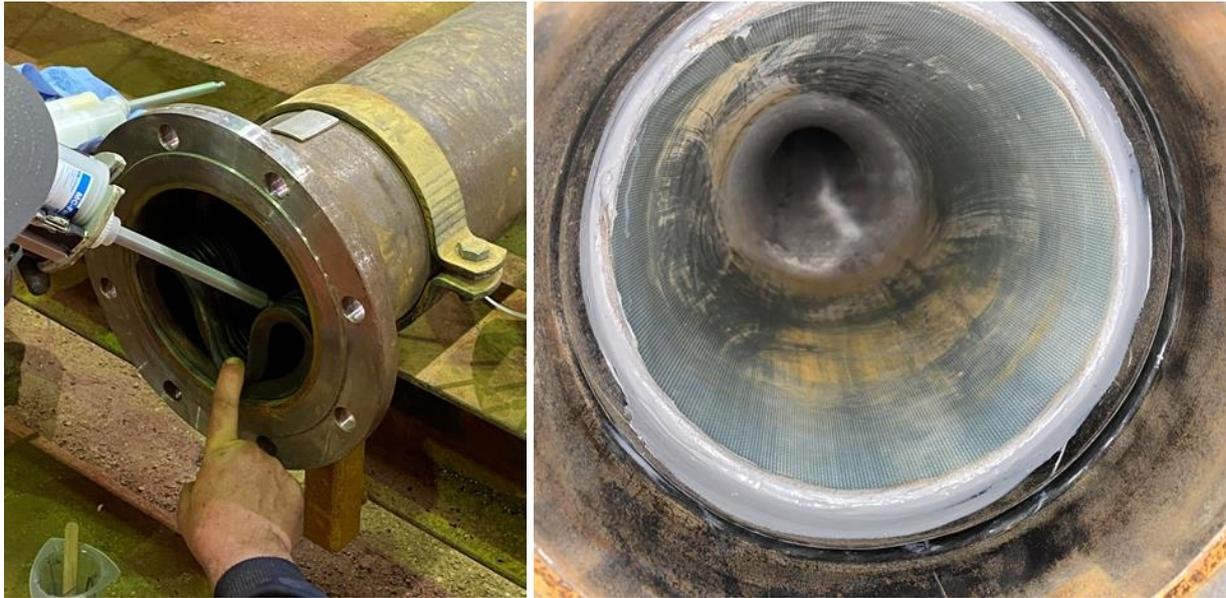
Figure 18. Replacing the sleeves with resin sealant on "Starline Structure-S": applying the sealant (left), rework result (right).
