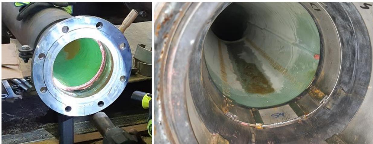
Figure 19. Replacing the sleeves with resin sealant on "Esders HPS Liner": application of sealant (left), rework result (right).
