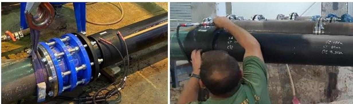
*Figure 40. PE flange/ electrofusion couplers: "egeLiner" (left) and "Compact Pipe" (right).*
