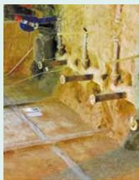
Rehabilitation task: Rehabilitation of three damage scenarios in each case in a liner-rehabilitated concrete main sewer (DN 300)
