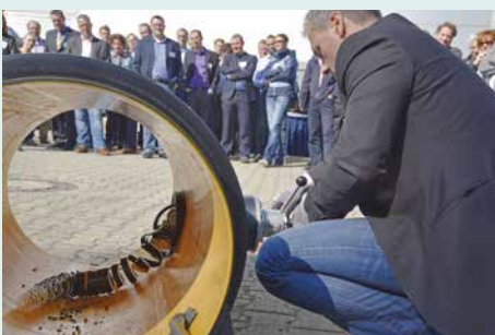
Practical demonstration: trimming off the projecting socket after welding a joint
