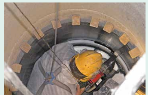
The joints between the individual elements are carefully sealed.
