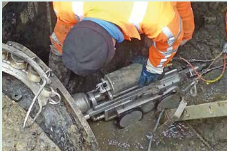
In-situ deployment of sewer radar
