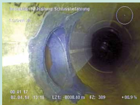
B: Tight lateral connection in the NF lined pipe
