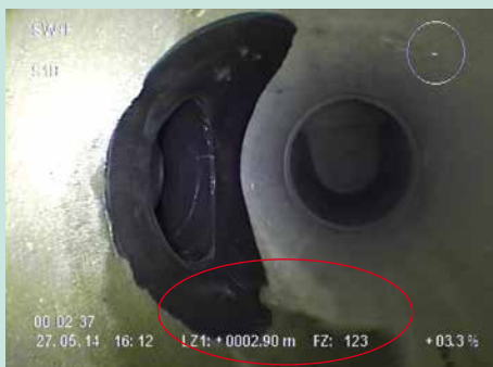
D: Moisture, with no infiltration, Example 2
