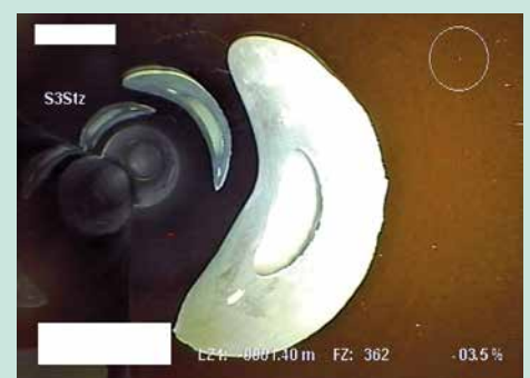
Figure 7: The best-graded lateral connection for the „Functionality“ criterion, after HP cleaning in each case; concrete pipe (left); vitrified-clay pipe (right)
