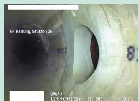
Figure 4: The best-graded lateral connection for the „Functionality“ criterion, in each case after HP cleaning; GRP lined pipe (left); NF lined pipe (right)
