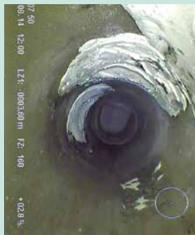
Figure 8: The poorest-graded lateral connection for the „Functionality“ criterion, after HP cleaning in each case; concrete pipe (left); vitrified-clay pipe (right)
