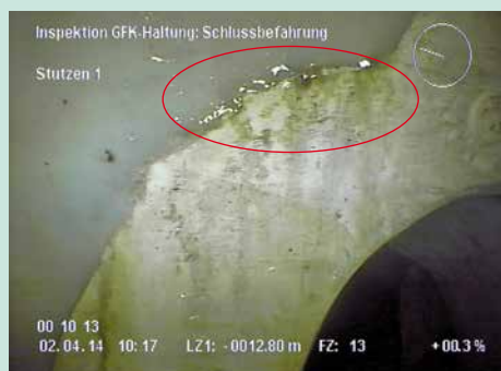
D: Moisture, with no infiltration
