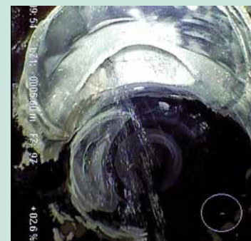
F: Leaking lateral connection in vitrified-clay pipe
