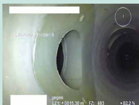
Figure 4: The best-graded lateral connection for the „Functionality“ criterion, in each case after HP cleaning; GRP lined pipe (left); NF lined pipe (right)
