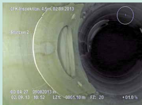
A: Tight lateral connection in the GRP lined pipe
