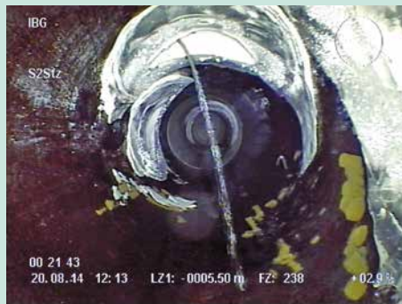
Figure 8: The poorest-graded lateral connection for the „Functionality“ criterion, after HP cleaning in each case; concrete pipe (left); vitrified-clay pipe (right)
