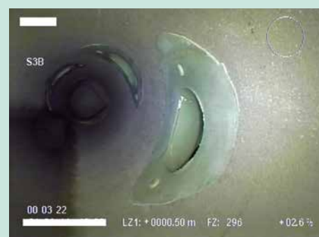
Figure 7: The best-graded lateral connection for the „Functionality“ criterion, after HP cleaning in each case; concrete pipe (left); vitrified-clay pipe (right)
