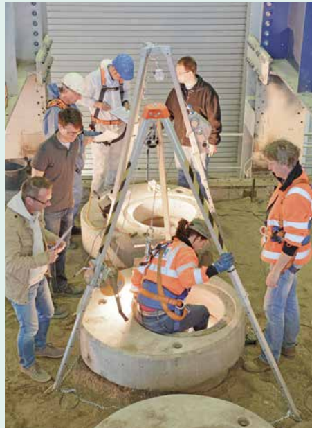
Acceptability of repair: the assessment committee subjected all the manholes to extremely precise inspection.
