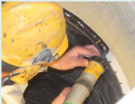
Test task: the participants had to repair a „pre-damaged“ manhole.
