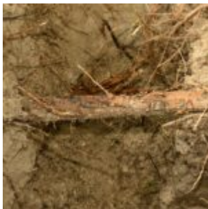
Horizontal root ingrowth in the pipe trench
