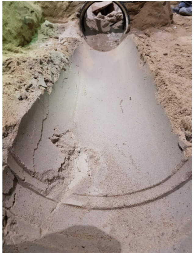
Pipe enclosure with minor defects (DN 300)
