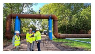
Bypass of 13,000 m<sup>3</sup>/h: Pumping stations and pressure sewer pipes to divert the flow from the rehabilitation stretch to ensure continues flow towards WWTP
