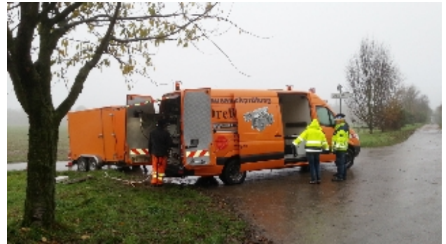
Field research: Inspection of a pressure pipe
