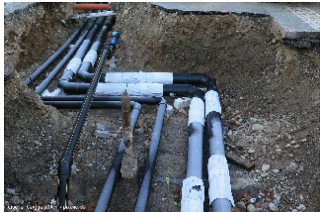
Open-trench installation of district-heating piping
