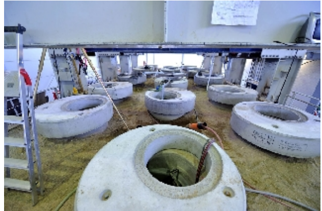
IKT's Comparative Test manhole renovation
