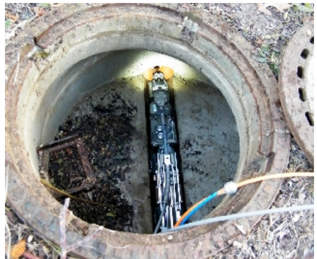
Sewer camera in use
