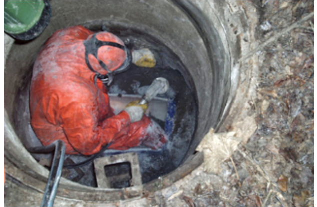
CIPP liner: Taking a sample in a manhole
