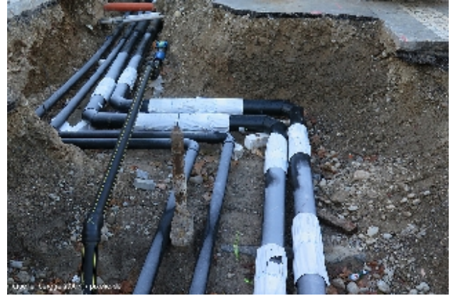
Open-trench installation of district-heating piping
