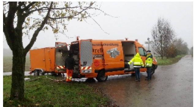
Field research: Inspection of a pressure pipe
