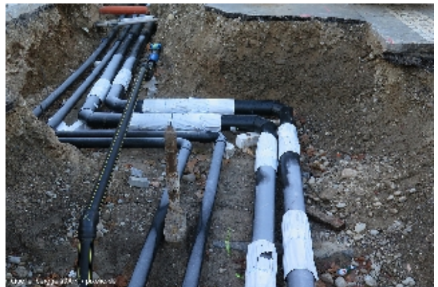
Open-trench installation of district-heating piping
