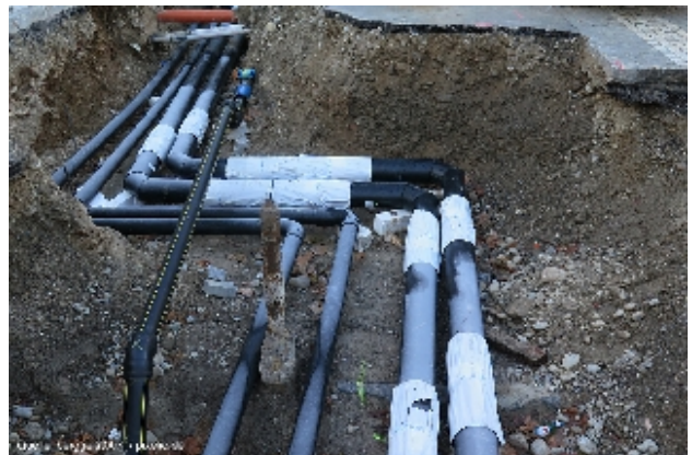
Open-trench installation of district-heating piping
