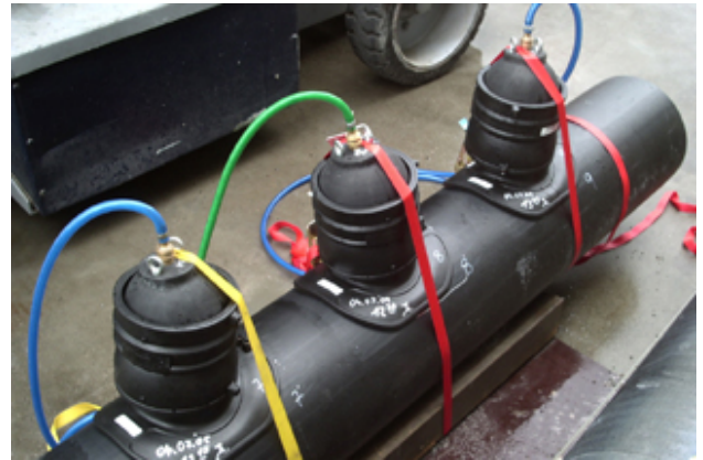
Testing sewer lateral saddles
