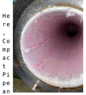
${\sf d}$  Clearly recognisable longitudinal fold in an installed liner
