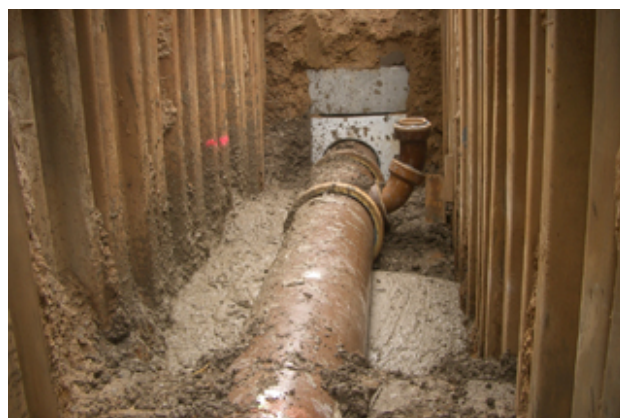
Well bedded, longer service-life
