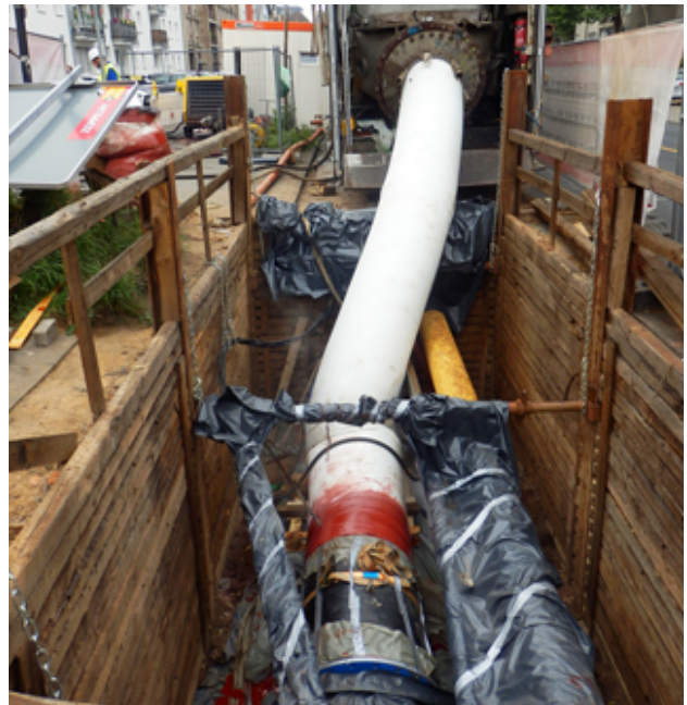
IKT Compare: testing lining systems for the trenchless rehabilitation of pressure sewers
