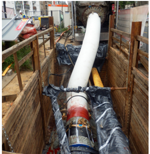
IKT Compare: testing lining systems for the trenchless rehabilitation of pressure sewers
