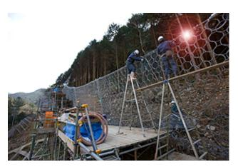
High tensile steel mesh barrier for rockfall protection. Energy absorption: 150hj, Height: 4m, Length: 65m
