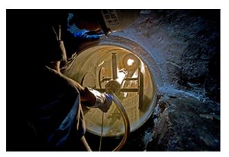
Sewer pipe rehabilitation with SEAMLESS LINER. Host pipe: DN600, Length: 70m; Wall thickness: 14mm
