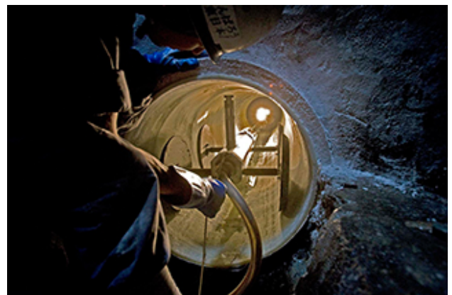
Sewer pipe rehabilitation with
