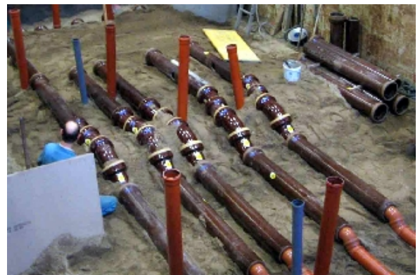
Construction of a sewer
