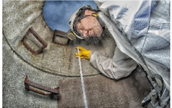
Manhole renovation Research
